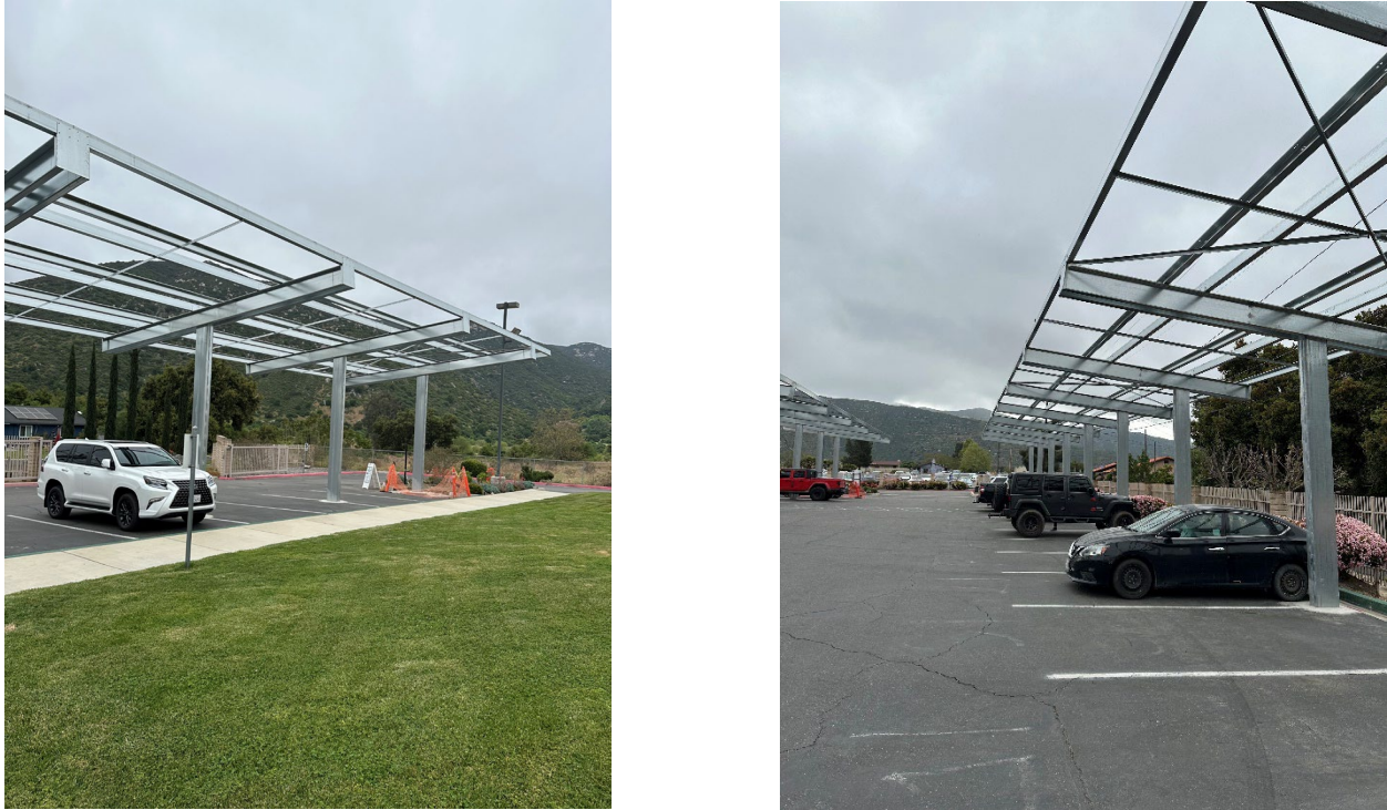
Figure 10. Progress Photo for the Rincon Clinic Solar Carports Project
