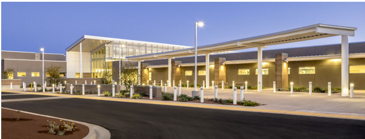
Figure 14. Fort Yuma Health Center
